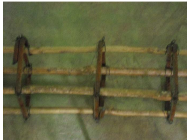
Figure. 2 - Bamboo as Reinforcement in Beam
