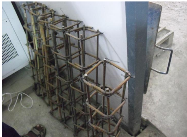
Figure. 1 - Bamboo as Reinforcement in Beam
