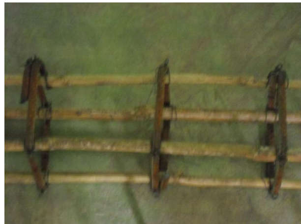
Figure. 2 - Bamboo as Reinforcement in Beam
